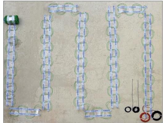
Example installation: simple design with spare heating cable and temperature sensors
